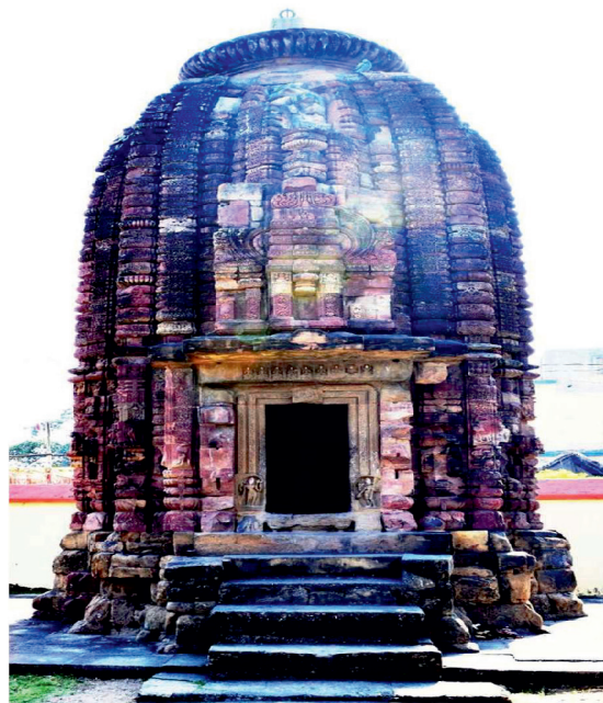
Fig. 2: General View: Siddheśvara Temple, Three Temple Complex, Boudh Town
